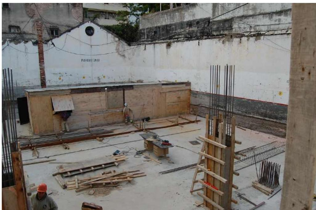
LOSA s/1ºSS COMPLETADA Y PRIMERAS COLUMNAS DE LOSA s/PB
